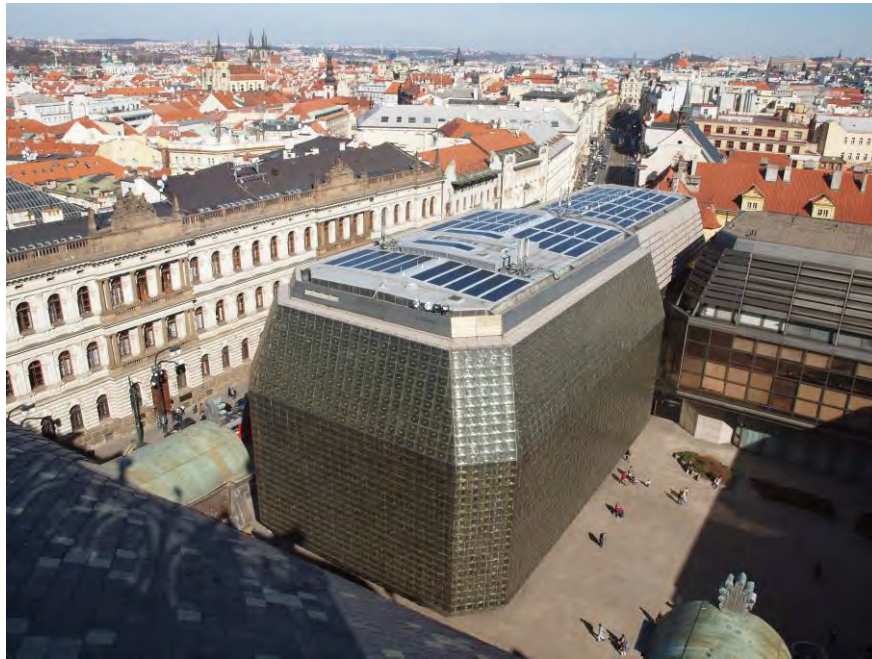
Figure 1. PV array on the Prague National Theatre - New Scene Building roof.
